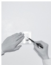
Mark drill holes using the jig.
