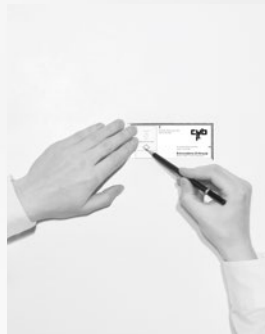
2. Mark drill holes with the drilling template.
